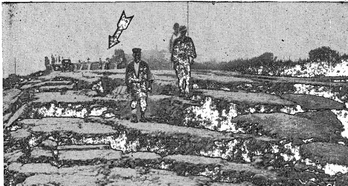
MOTHER EARTH'S TERRIBLE FORCE . . . The devastating wrath of an earthquake is clearly depicted in this scene outside Fukui, Japan. Civilians tread like pre-historic men over the newly formed earth and large crevices which were left when the section was rocked by forceful quakes. In the distance (marked with an arrow) is a highway bridge which was pushed upwards and raised several feet higher by the quake. The earthquake, worst peacetime disaster to date, left a death toll of more than 3,000 persons. Now comes the job of reconstruction. The Red Cross at present is caring for and feeding hundreds of thousands left injured and homeless by the catastrophe.
